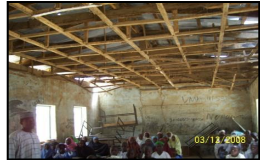
Figure11: Picture of a classroom showing the structure without ceiling-sheets in Kano.
