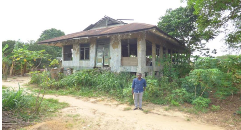
Fig. 1: Showing old Ahoada District office
