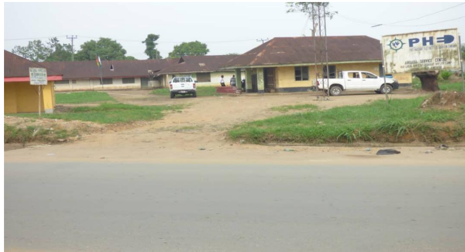
Fig. 2: Showing Ahoada District structures, now been used as office of PHED
